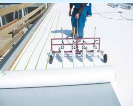
applying the roof sheet adhesive
