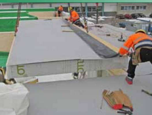
installing of prefabricated roof elements
