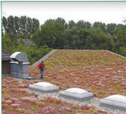
grassed roof system with AUSTROPLAN TPO roof liners
