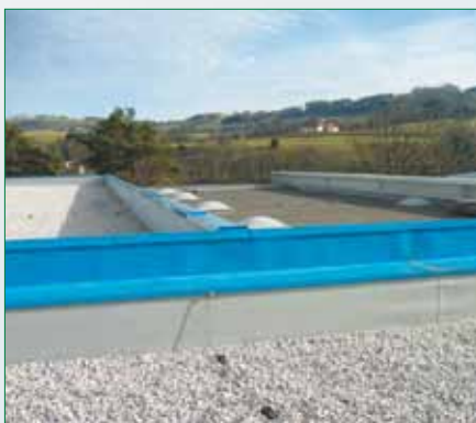
reorganized business building with AUSTROPLAN TPO roof liner sealed
