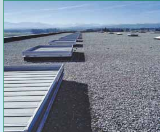
gravel ballast roof systems
