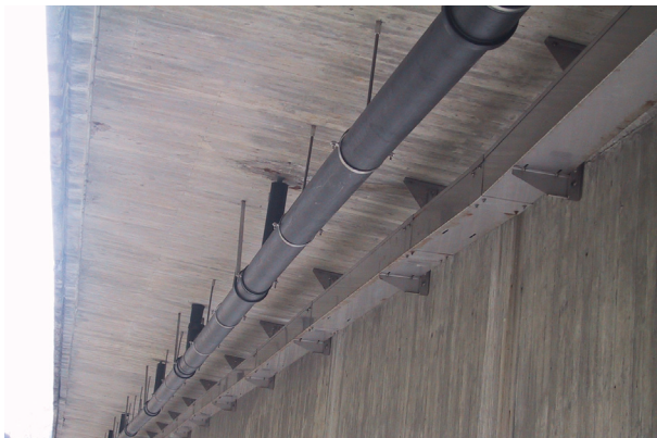
Figure 8: Side drainage system.
