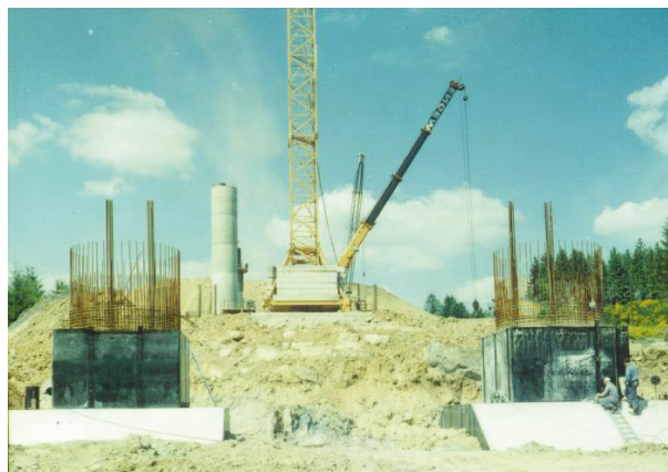
Figure 3: Cast in Situ-installation method.
