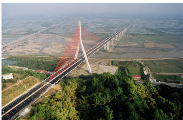
Figure 14: PE-pipes for protection of bridge stay cables.
