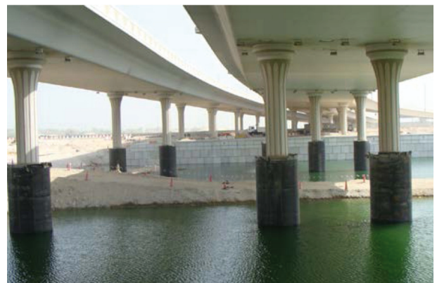
Figure 6: Bridge piers protected by AGRU Sure Grip® concrete protective liners.
