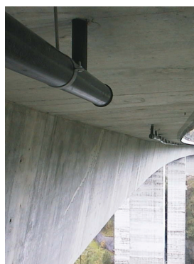
Figure 9: Listertalbrücke A10 Tauernautobahn drainage system.
