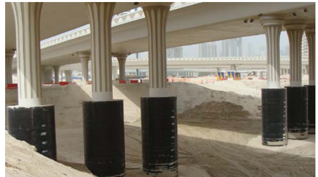
Figure 2: AGRU Sure Grip® concrete protective liner seal and protect concrete foundations.
