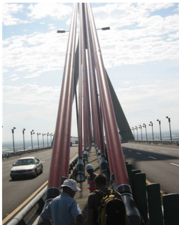
Figure 14: PE-pipes for protection of bridge stay cables.
