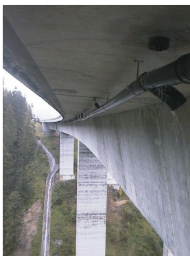
Figure 9: Listertalbrücke A10 Tauernautobahn drainage system.
