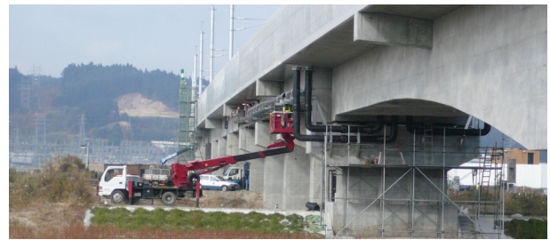
Figure 11: Installation of the PE 100 sprinkler system.
