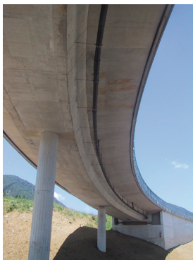
Figure 7: Middle drainage system.
